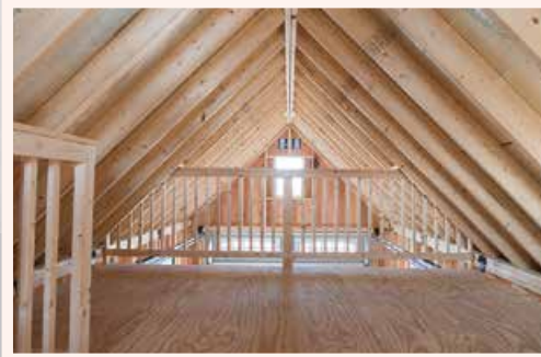
Interior of Keystone Garage (optional loft & railing)
