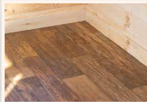
Loose Lay Linoleum on Floor
